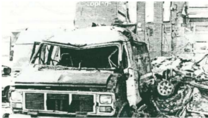
Destroyed car at about 40 m from the explosion [3]
