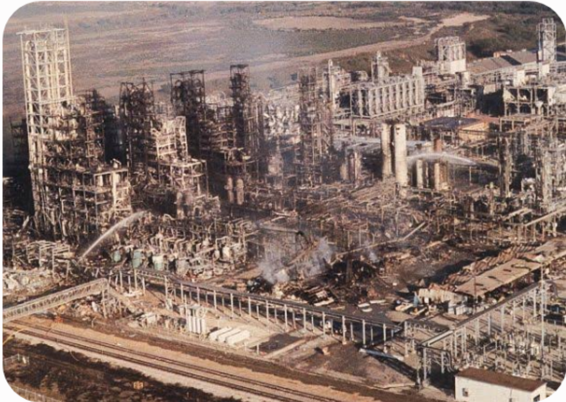
The devastated process structures at the Pasadena plant. Source: The Pop History Dig
