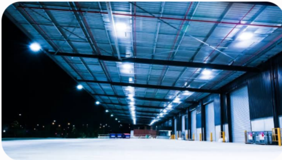
Properly shielded high-bay lighting setup reducing direct glare on the factory
